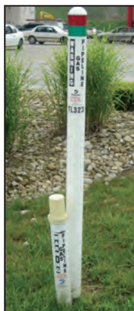
2. Linemarker and cathodic protection test station
