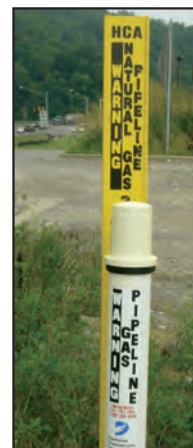
5. HCA marker and cathodic protection test station
