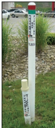
2. Linemarker and cathodic protection test station
