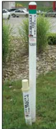
2. Linemarker and cathodic protection test station
