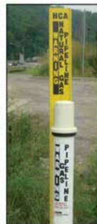
5. HCA marker and cathodic protection test station
