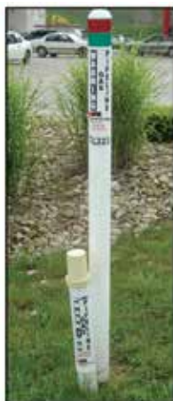
2. Linemarker and cathodic protection test station
