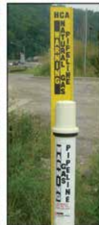
5. HCA marker and cathodic protection test station
