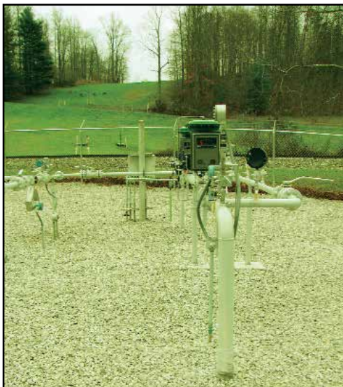
This pipeline brings in natural gasoline to a loading rack for rail transportation. The cleared area in the background is a right-of-way for the natural gasoline pipeline. Signs for recognizing a leak within a right-of-way are listed in the text above.
